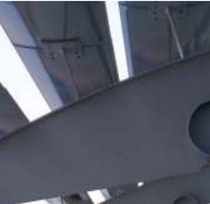
Custom blade supports. The custom blade supports shown have been specifically designed for cantilevered projections of Audi showrooms. csairfoil AF270 blades are fixed onto vertical custom-made supports, attached to horizontal support segments. The lightweight but extremely robust structure of csairfoil blades allow for the design of any imaginable support, fixture, suspension or attachment, proving to be an extremely versatile, architectural design element and sun control system at the same time.
