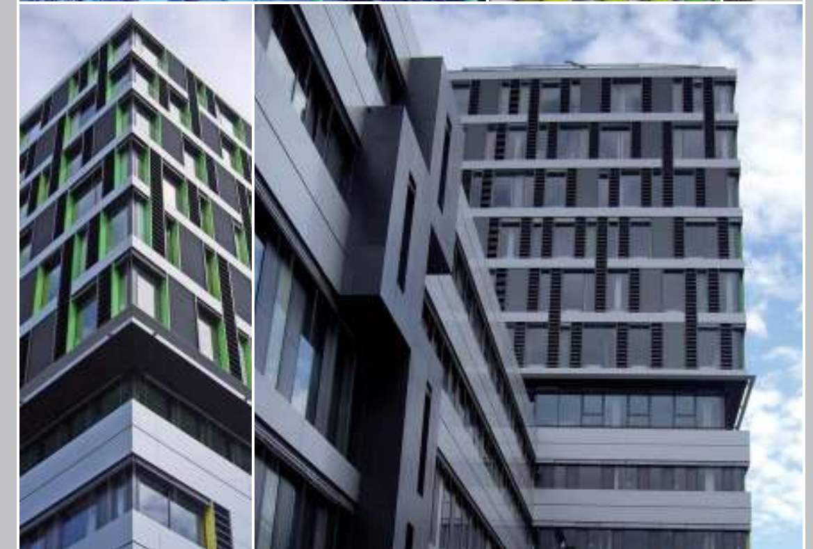
Project Landratsamt Heilbronn: Colour LEDs integrated into the embrasures of windows illuminate at night horizontally arranged noise-absorbing CS Airfoil AF320 LB solar shading blades to make the illuminated building also at night a focal point of attention.
