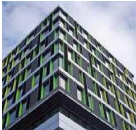
▲ Office building. The horizontally mounted c|sairfoil® noise-absorbing blades AF320 LB offer efficient solar protection and reduce external noise contamination getting into the inside of the building.
