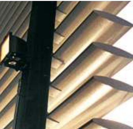
Birdsmouth brackets. Horizontally mounted csairfoil AF270 blades are shown from behind the facade of a building. Birdsmouth brackets had been fixed onto vertical support segments at specified distances and csairfoil blades were simply slotted into the brackets and fixed with screws or rivets. Birdsmouth brackets allow for speedy onsite installations and have the additional advantage of being virtually invisible when seen from the front.
