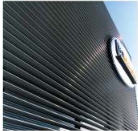
▲ Cinema. Horizontally mounted c|sairfoil® blades AF270-F cover the facade of the building.
