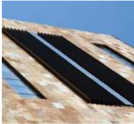
▲ Office building. Vertically mounted c|sairfoil® AF200 E blades cover the emergency staircase.
